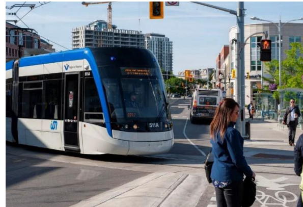
Figure 3-5 ION Line Light Rail, Waterloo
